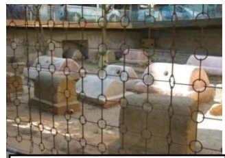
Via romana Plaça Vila de Madrid Renovation work and museum project in progress
