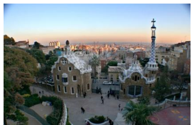
Park Güell New museum project "Gaudí, the park and the city", work in progress
