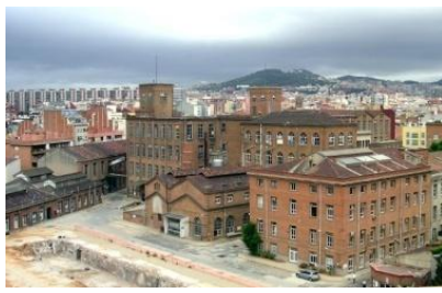
Fabra i Coats Work, neighbourhood and the city Renovation of the power systems + work interpretation centre, phase 1, with the participation of the social fabric
