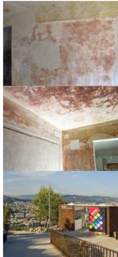
Restoration of the interior walls of the Officials' Pavilion, 2014-15.
