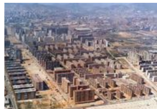
Early in the 1960s, many shanty dwellers from Montjuic settled in the public housing estate of Sud-Oest Besòs. The residents began to pay for their flats, owning them after 30 years. In 1990, the large empty avenue was converted into a very attractive promenade, Rambla Prim. © Patronat Municipal de l'Habitatge de Barcelona.
